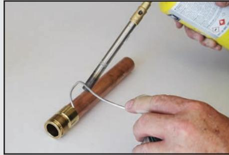
Solder the brass adapter to the copper pipe. Allow the fitting to cool.
