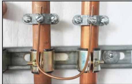
Install a ground strap. (Not included.) When installing a Purearth2o Water Conditioning System, the ground wire may be interrupted and therefore you must install a ground continuity strap.
