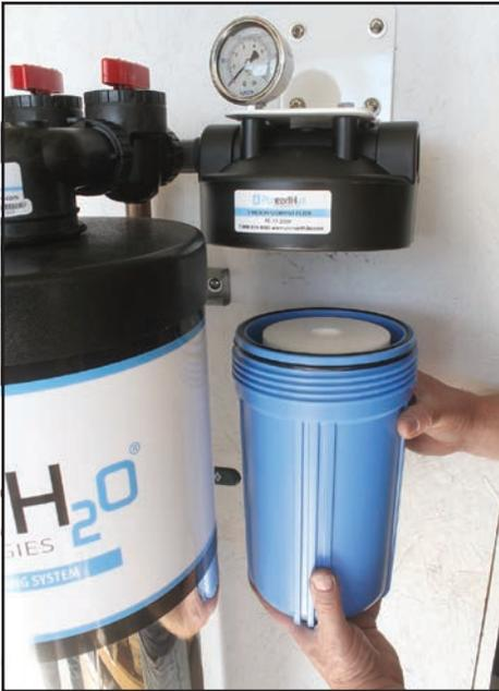
Insert the 5-micron filter into the filter housing.
