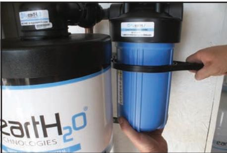
Tighten the filter housing with the tool supplied.
