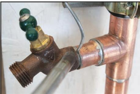
A hose bib and a ball valve **MUST** be installed on the outlet side of the pipe before it goes into the house. This is the only manual way to clean the media and prevent black carbon water entering the house. (This is **VERY** important and required in order to clean the carbon media inside the tank)
