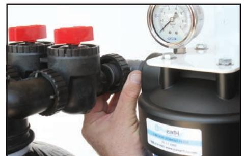
Mount and screw the filter housing to the wall and tighten 1" PVC fitting to the bypass valve.
