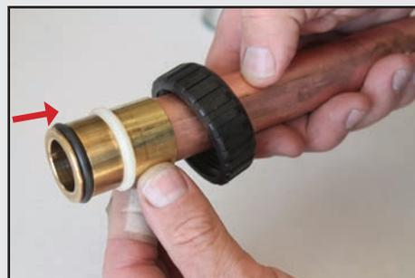
After the fitting has cooled, slide the nut (black) on first, then the split ring (white), and finally the O-ring (black).
