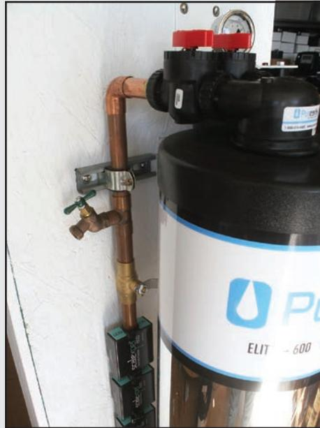
Cut and remove a section of the water supply lines where the system is going to be installed. Install the system after the pressure regulator. The location of the water conditioning system should be level and located nearest the pressure regulator.
