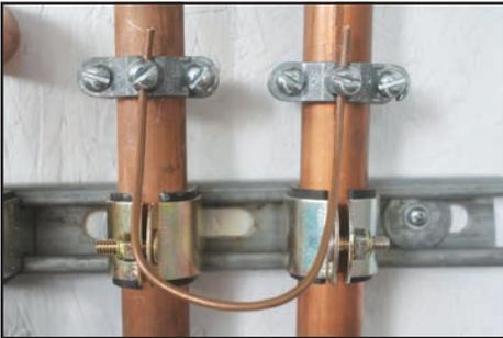
Install a ground strap. (Not included.) When installing a Purearth2o Water Conditioning System, the ground wire may be interrupted and therefore you must install a ground continuity strap.
