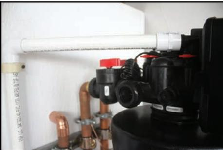
Follow all state and federal plumbing codes when installing the drain line. Install an "air gap" at the end of the drain line. Do not connect directly to a sewer line.
