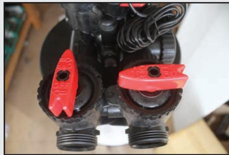
Turn on the inlet side of the bypass valve to service position. Do not turn on the outside of the bypass (should remain in bypass position.) Slowly fill the tank.
