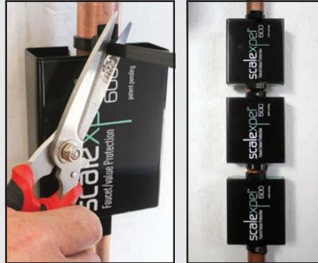
Installation of the Scalexpel Protection units will take place on the outlet side of supply pipe. Install units on a area of straight pipe, 20" long if possible. Secure with the supplied plastic fasteners. Install units from top to bottom.
