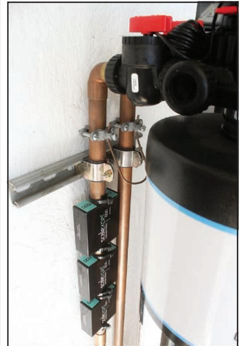
Cut and remove a section of the water supply lines where the system is going to be installed. Install the system after the pressure regulator. The location of the water conditioning system should be level and located nearest the pressure regulator.
